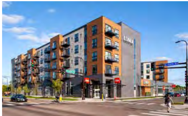
LOWA 46 - MINNEAPOLIS, MN
